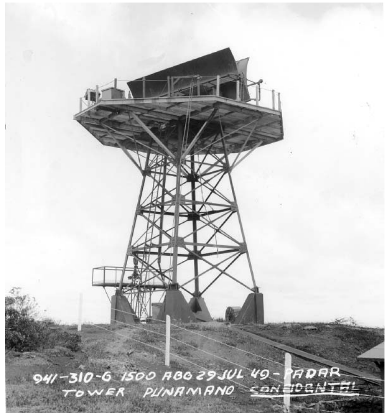
AN/CPS-1 microwave search radar antenna at Punamao AFS July 29, 1949. The last Air Force unit to man the station was the 614th Aircraft Control and Warning Squadron on December 11, 1948. Base camp was located across the highway from Kahuku AAB. (Photo from the 15th Air Wing History Office)
