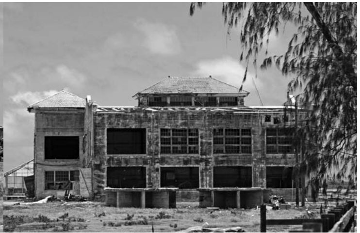
Rear of the old Marconi/RCA Transmitter building in 2010; two raised platforms in the foreground once supported liquid storage tanks. (Photo by the author)
