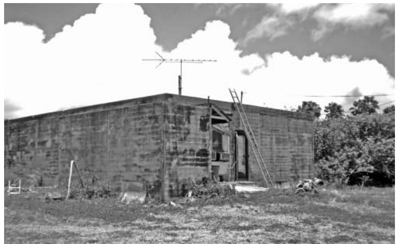
Kahuku AAB Telephone Exchange building in 2010. (Photo by the author)
